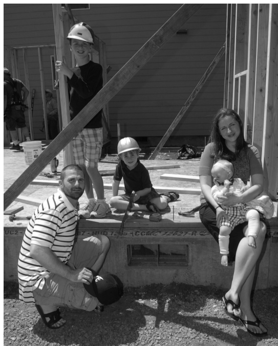
While visiting the worksite, the Ambrose family posed for us on the foundation of what they soon will be calling home. From left to right: Daren, Iverson, Isaac, Lila, and Lisa.
