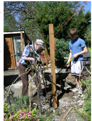
David James and a Marist High School student setting fence posts.
